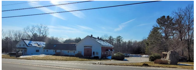
640 Maple Street, Contoocook, NH, An 1880 farmhouse on 5.5 acres near Exit 6, 189 that was converted into eight residential units.
